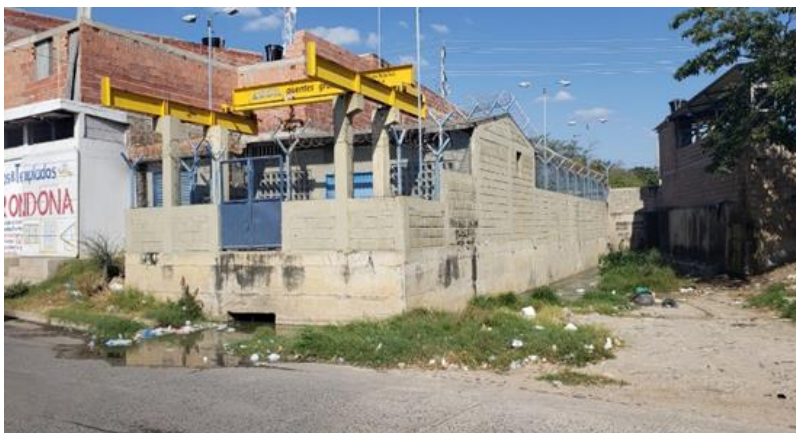
Figura 14. By pass Carrera 7H calle 19
